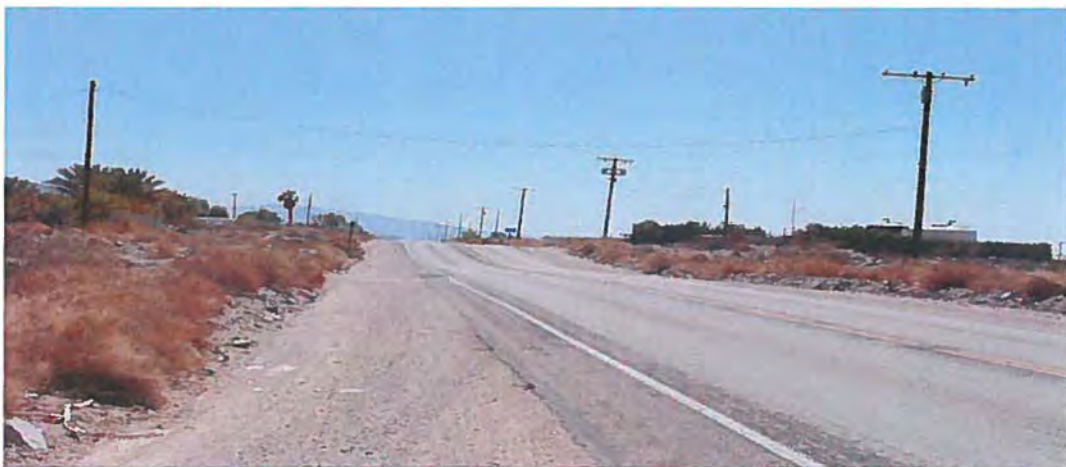
Looking East – Dillon Road Proposed Transmission Main Alignment; Booster Stn. 04701 on Right
